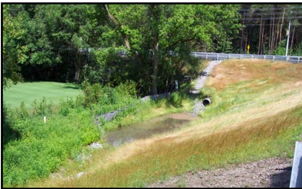
Illustration of a location where a noise barrier would not be effective.
